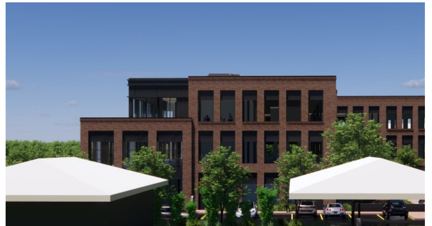
View of West Elevation
